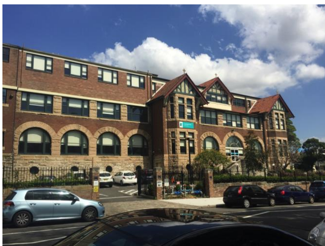
Figure 9 Former Lewisham Hospital site along West Street (to the north of the site)
